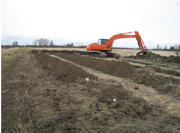
SC3 100.000 With 800 Ft Infiltrator 36" wide was installed over a mound that was created under II World War.
