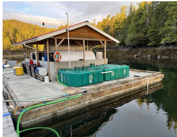
System connected in and out with green 2" hose, out have 30 Ft with weights to keep it down.
