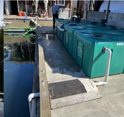
SC2F 1600 System ready for shipping via barge to Prince Rupert BC. On concrete barge connection with 2"
